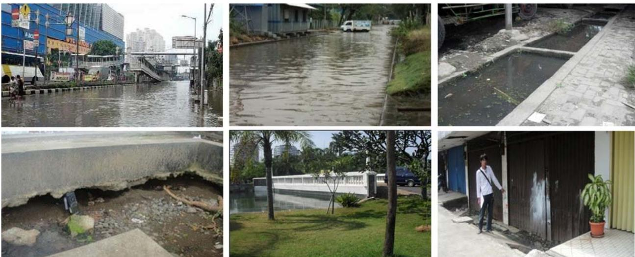
Fig. 9. The impact of land subsidence in Jakarta, e.g., tidal inundation “rob”, crack on infrastructure, the “sinking” bridge, problem in drainage, and problem of low level on the house to the road.
